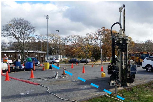
FIGURE 7. Demonstration test PRB implementation (blue line illustrates PRB).
