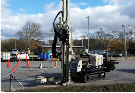
Figure 5 Geoprobe injection of Demonstration PRB on Cape Cod
