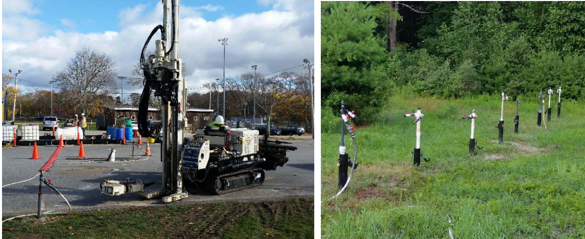
Figure 4. Direct-push drill rig used to advance temporary injection points for a PRB, and injection PRB using PVC injection wells.
